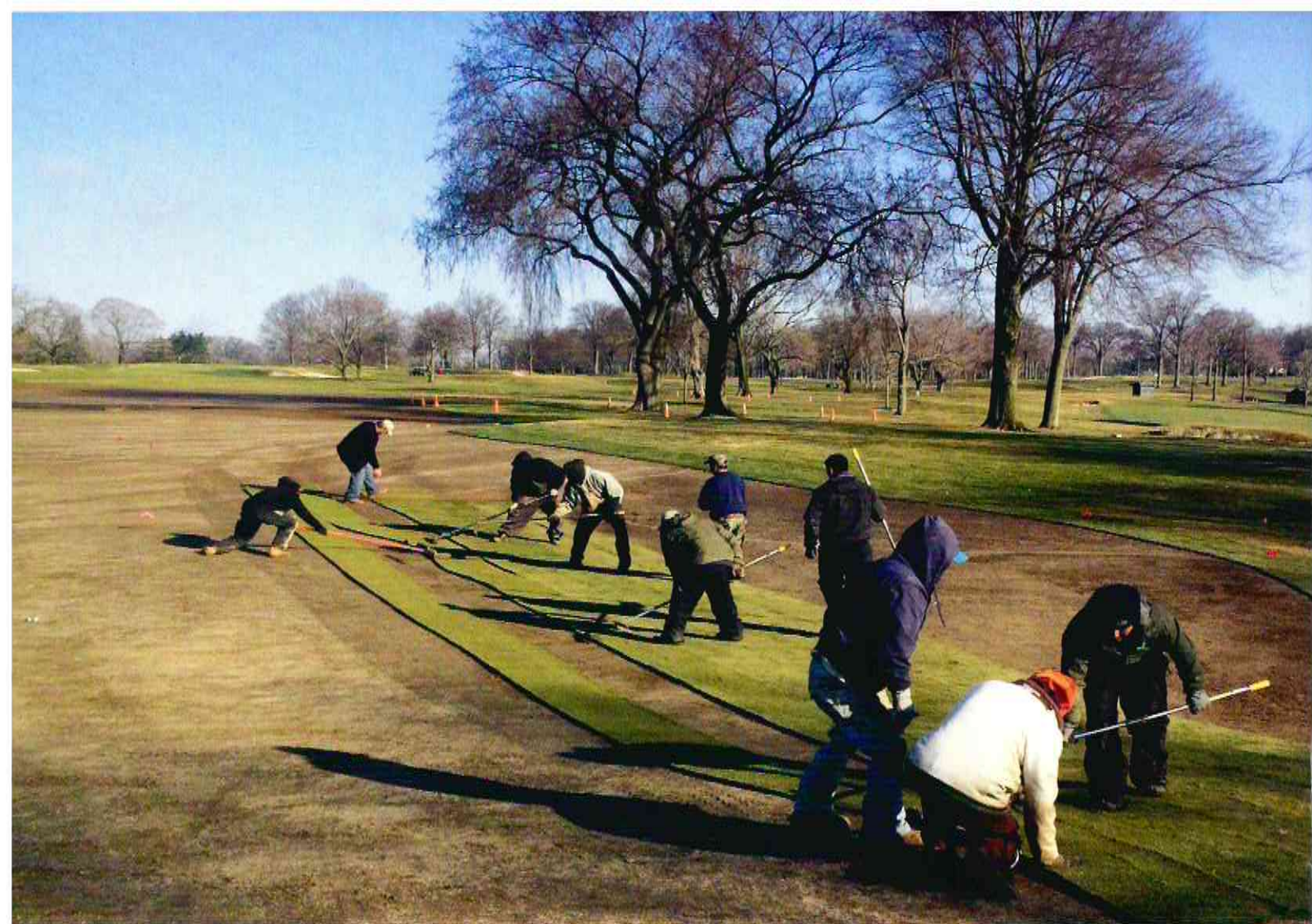
ABOVE: Laying sod at Morris County GC.
